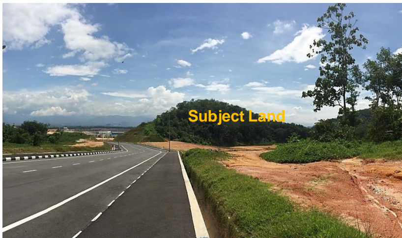
Access road to the Subject Land
