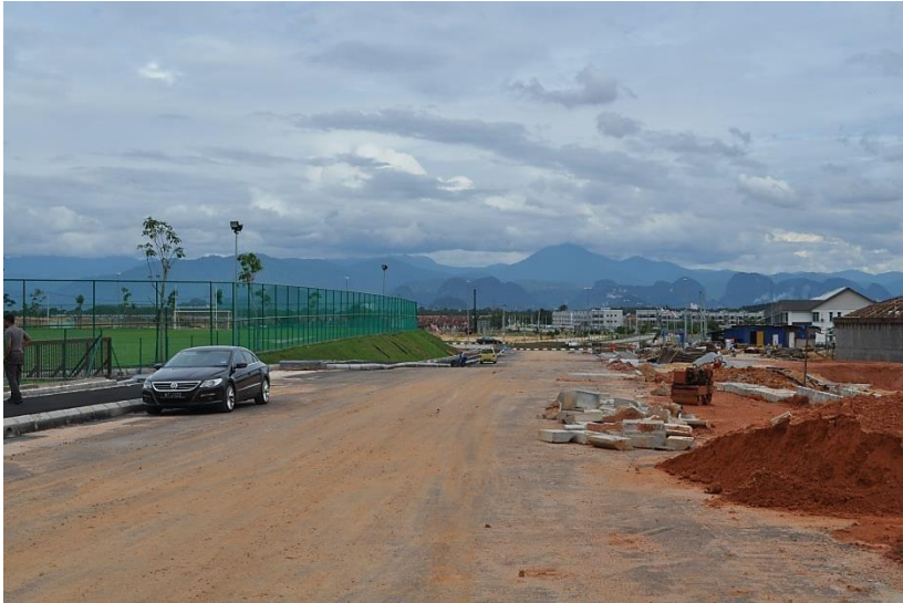
Access road to the Subject Land
