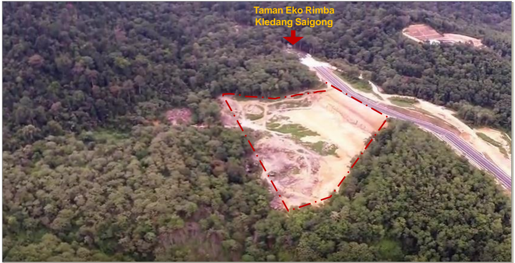
Aerial View of Subject land
